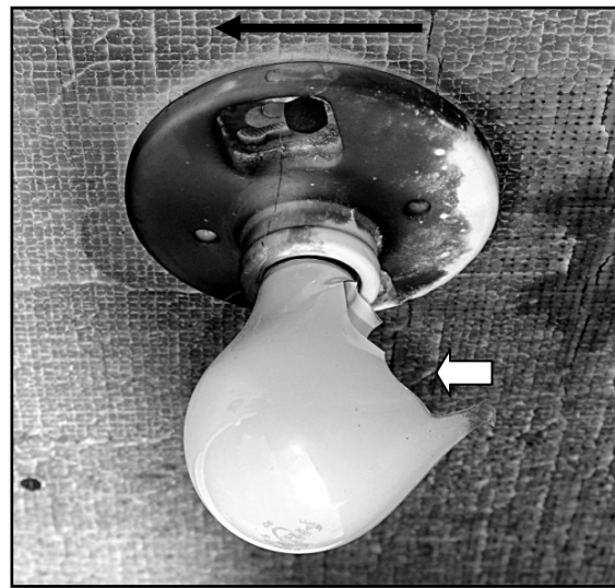
Figure 10. "Popped" bulb. Position C2, in ceiling jet.
